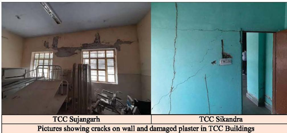
PMO Sujangarh observed cracks on walls and damage to the plaster in the newly constructed TCC building in November 2015 i.e. few months after
